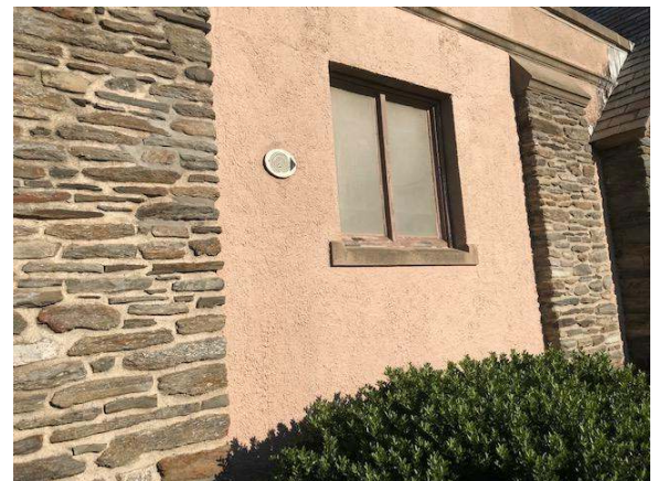
Touch-up of outside wall
